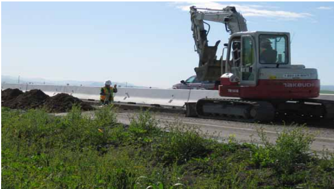
Paving digging Stage 2 traveled way
