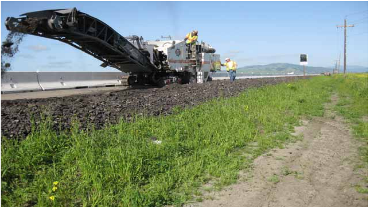
• Grinding @ Shore Rd
