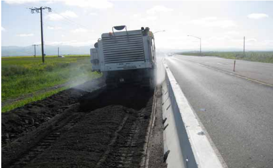
Grinding the widening at Shore Rd.
